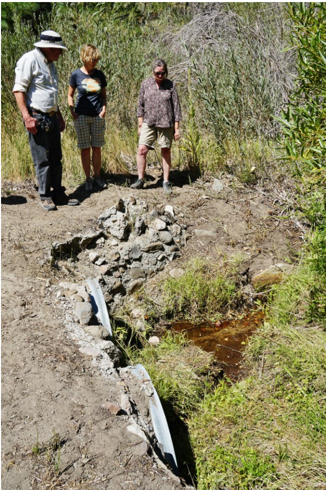
Site of the old Coyote Mill and present day culvert.
